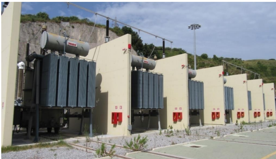
Figure 5.3: Firewalls – Shunt reactors
