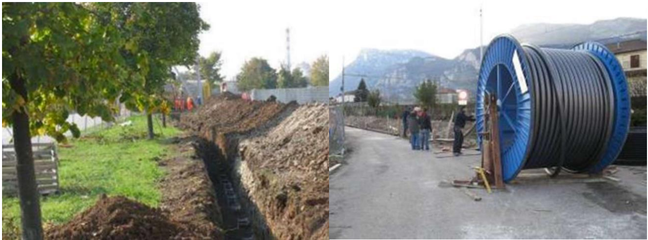
Figure 5.8: Example of cable laying in a trench
