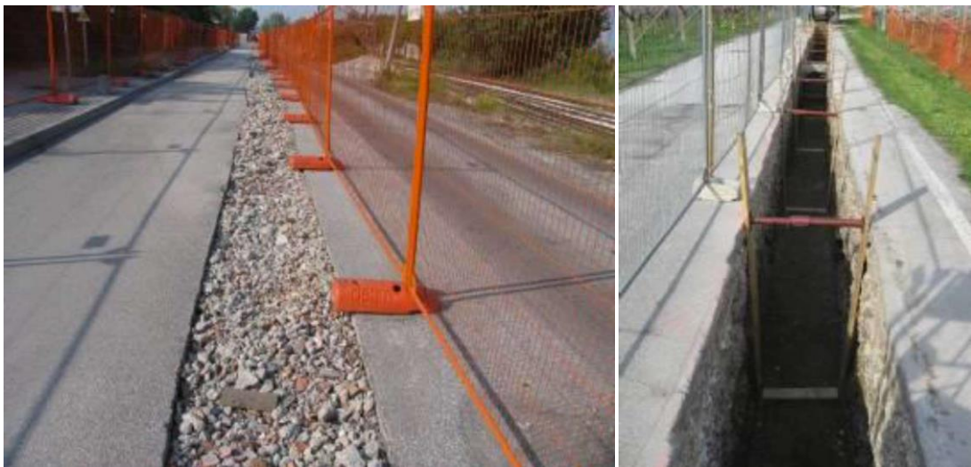
Figure 5.7: Example of cable installation on a paved road
