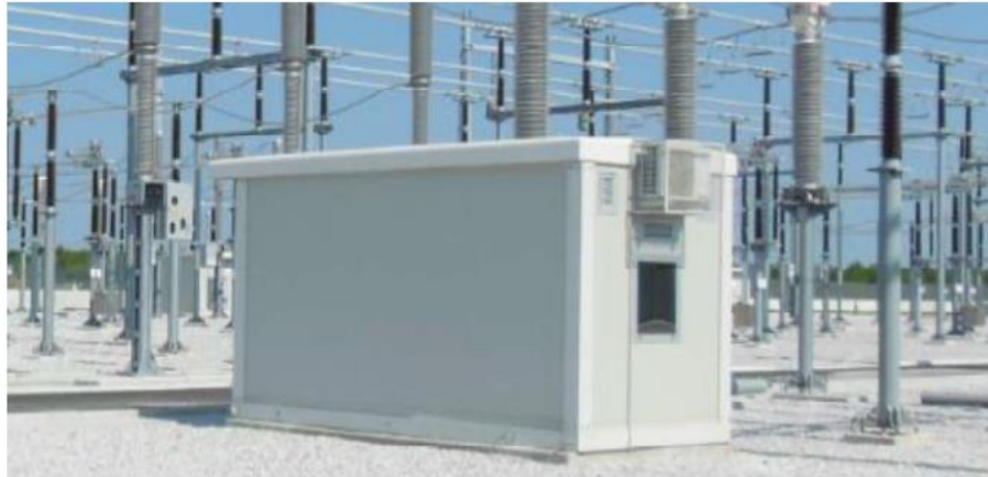
Figure 5.2: Prefabricated kiosk
