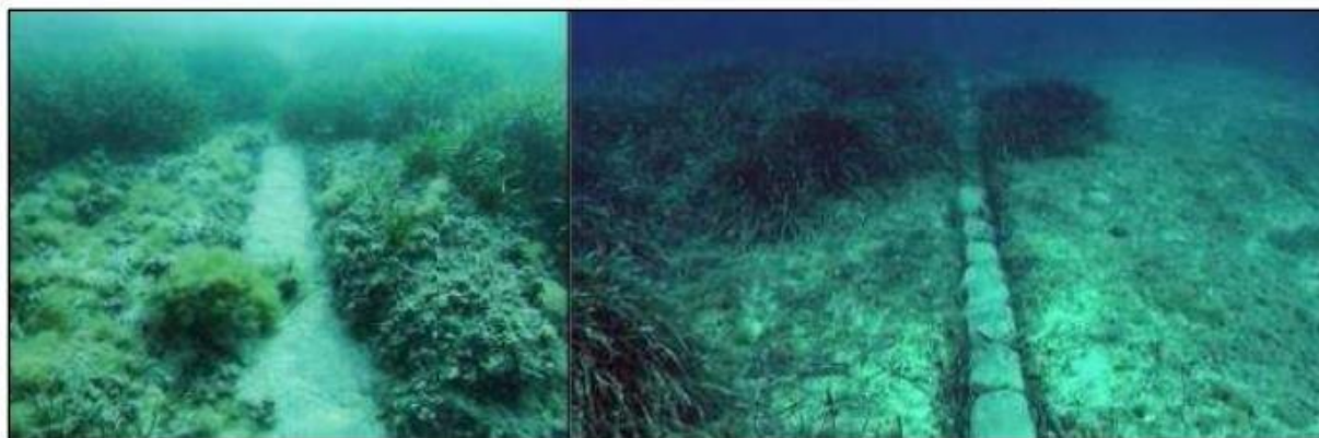
Figure 5.22: Trench over Posidonia on sand generated with a jetting machine
