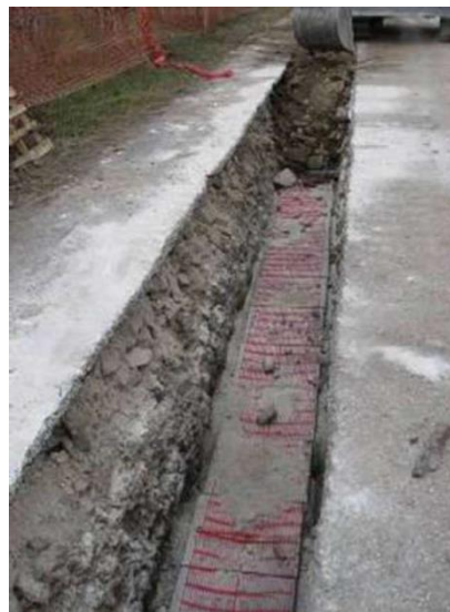
Figure 5.9: Backfilling with installation of protection plates and PVC mesh
