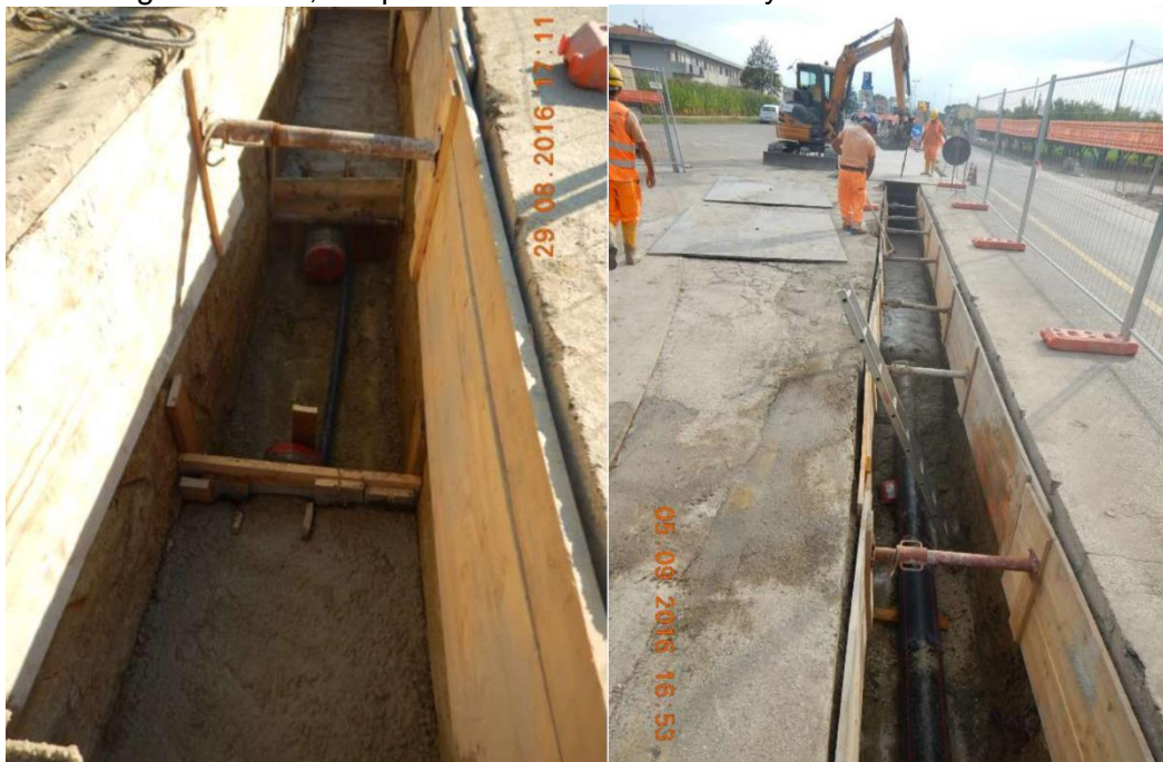
Figure 5.10: Power cable installation in HDPE pipeline
