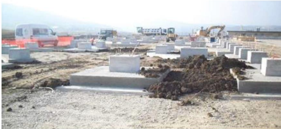
Figure 5.1: Single-core equipment foundations
