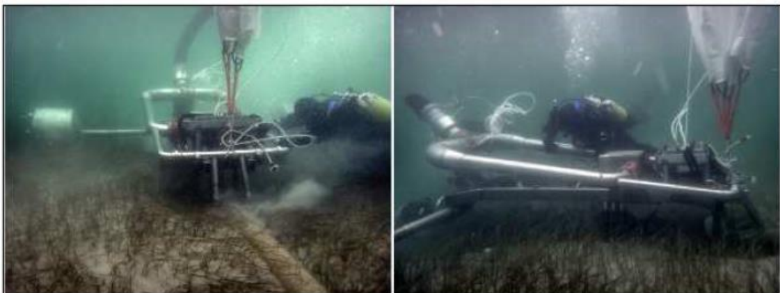
Figure 5.21: Machinery for jetting over Posidonia oceanica on sand sediments
