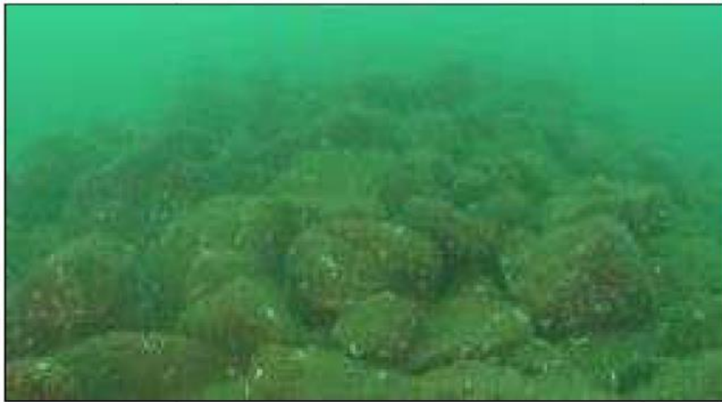
Figure 5.29: Cable cover by rock dumping
